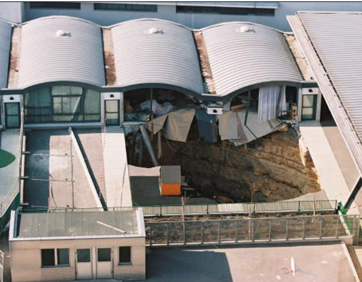
Figure 1.2 Cuvette de tassement 3D (Leblais et al. [1995])
