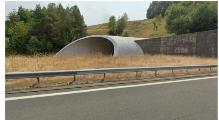
Tunnel de Montjeziu A75
